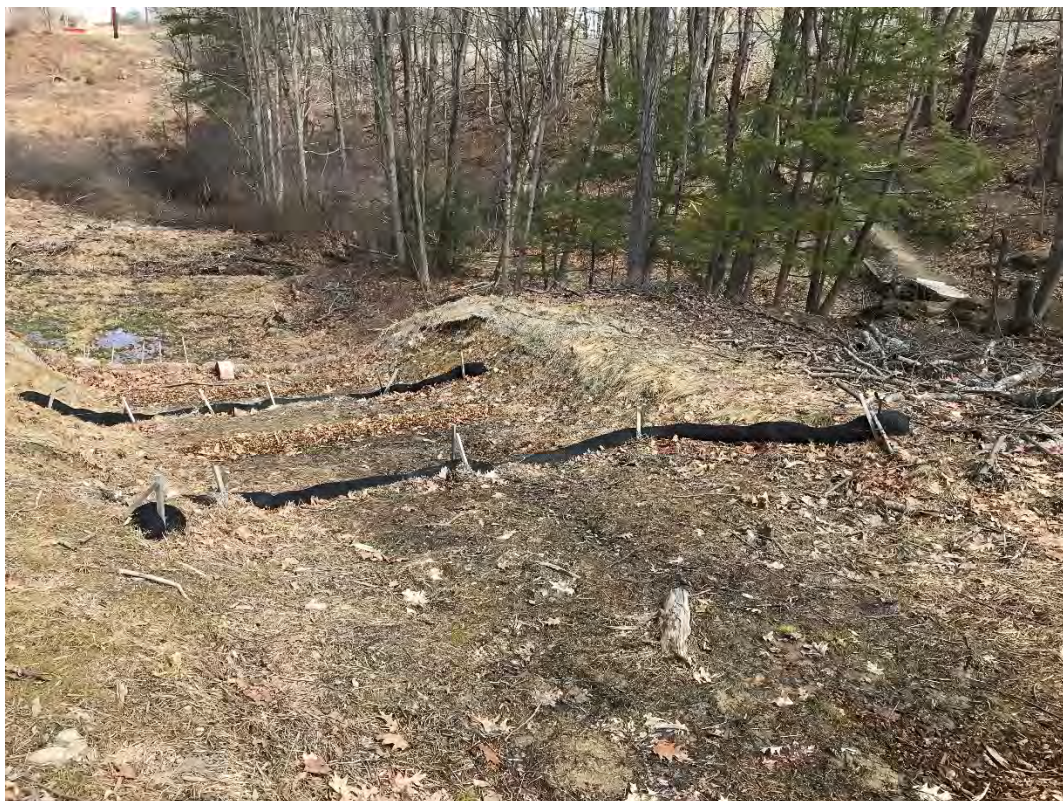
Fig 8: Lower portion of slope between Strs. 28 and 29. Viewing northeast. (03-29-21)
