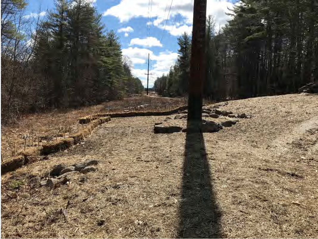
Fig 5: Str. 89 work area. Viewing southeast. (03-29-21)
